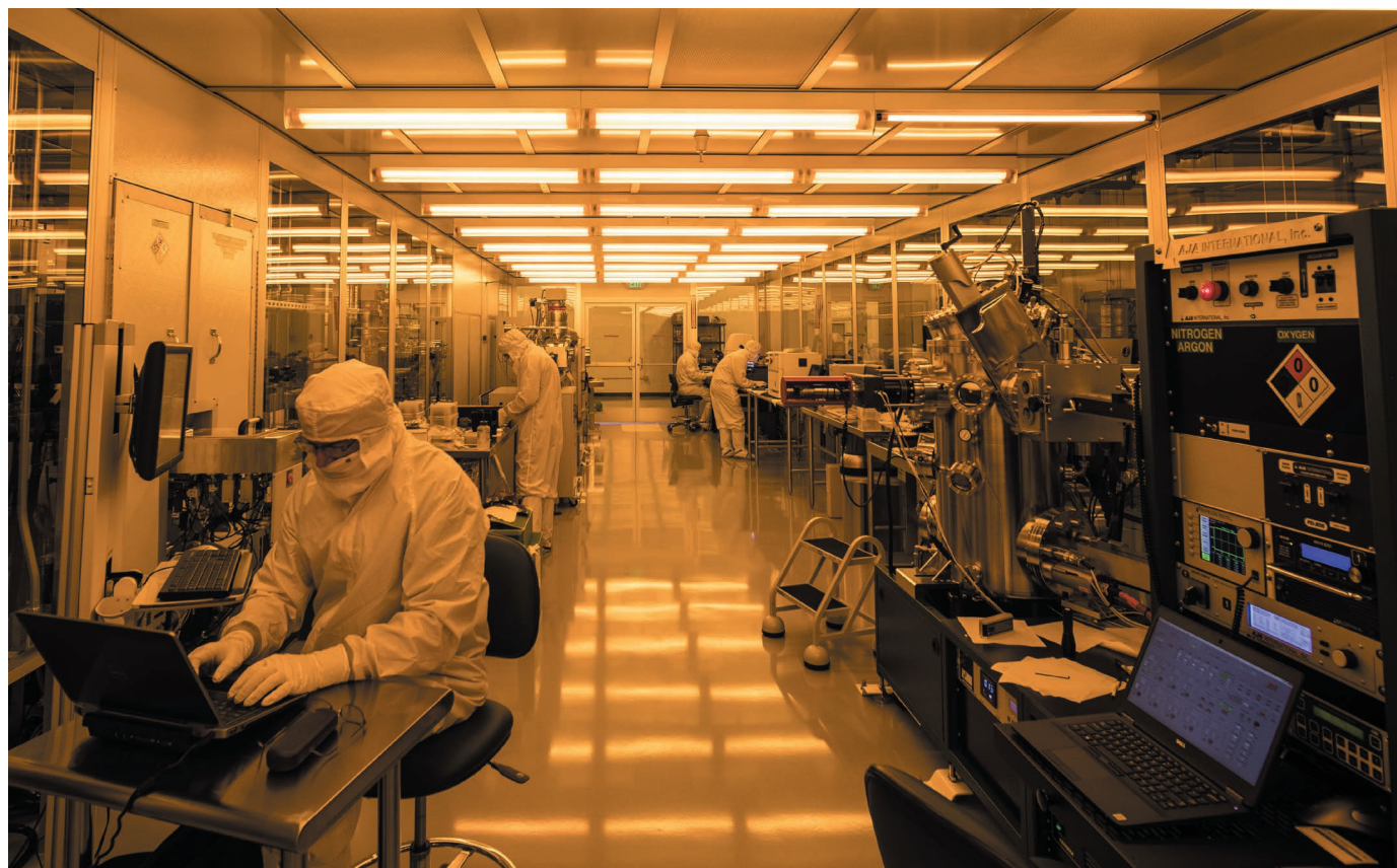
Inside the clean room at Rigetti Computing's Fab-1 facility in Fremont, California.
