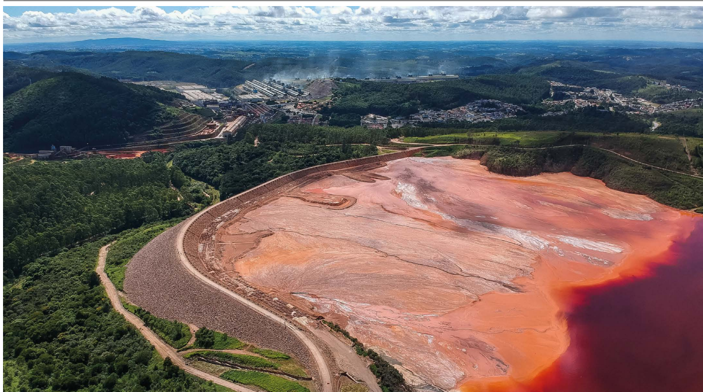
Figure 1 | A reservoir of 'red mud'. This dam near the town of Alumínio, Brazil, contains 25 million cubic metres of hazardous waste from aluminium production.
