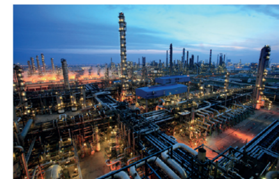
APC&RTO technologies of ECUST are applied at Sinopec & Petrochina (Pictured at Sinopec Zhenhai Refining & Chemical)
