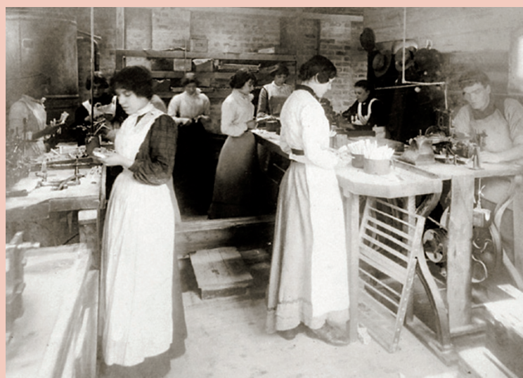
'A drilling shop. Boring tooth brush handles.' W. R. Tilbury & Co, Brush Manufacturers, Hackney, London, England. With thanks to BDA Museum.
