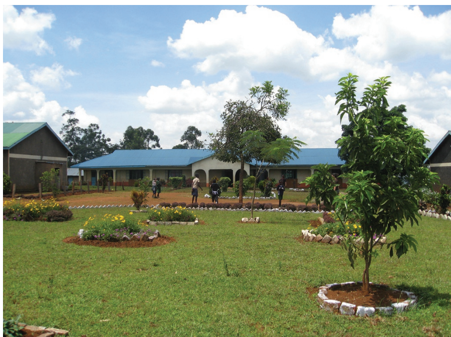
Fig. 1 The resource centre at the Akhonya Trust Children's Home which will contain the dental unit
