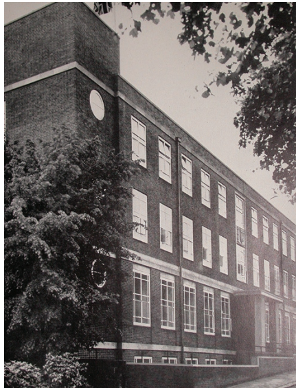
Fig. 7 The newly completed Charles Clifford Dental Hospital photographed before its official opening in October 1953
