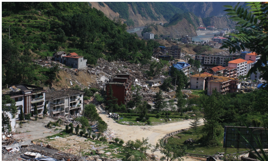
Fig. 1 A general view of the earthquake-hit Beichuan county, which is located in the northeast of the epicentre of Wenchuan county, Sichuan province. The view shows the concrete structures crumbling to rubble under their own weight, or being crushed by landslides
