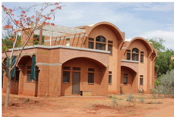
Fig. 3 A residence in Auroville constructed using compressed earth blocks
