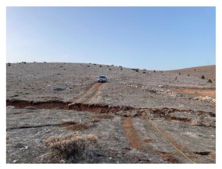
Fig. 2 Surface ruptures caused by the 2023 Kahramanmaraş Earthquake Sequence. Dirt roadway offset near the epicenter of the Ekinozu earthquake. Photo by Sinan Akciz, California State University, Fullerton.
