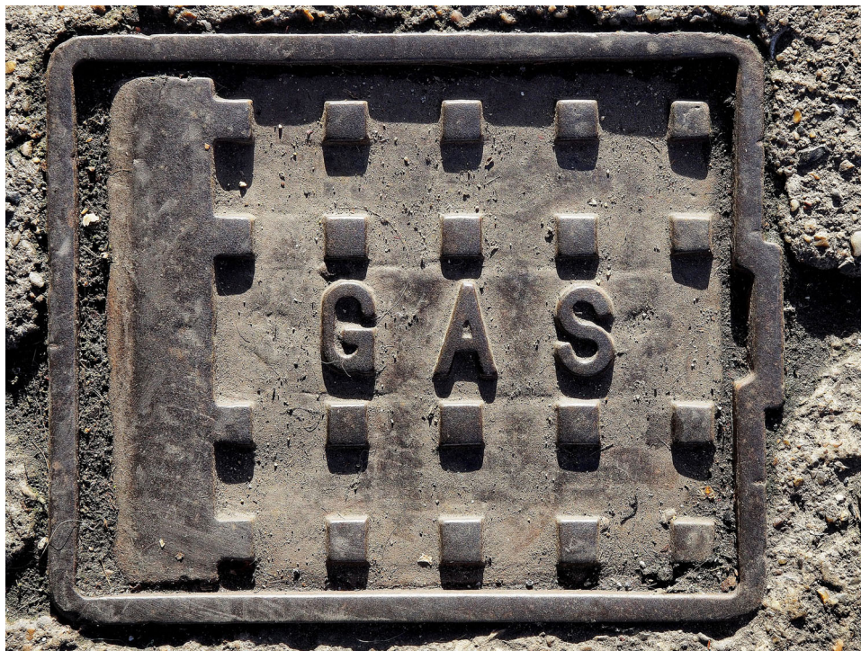
Fig. 1 Gas manhole cover. The fossil fuel industry is a major anthropogenic source of methane. Credit: Andrew Martin, Pixabay.
