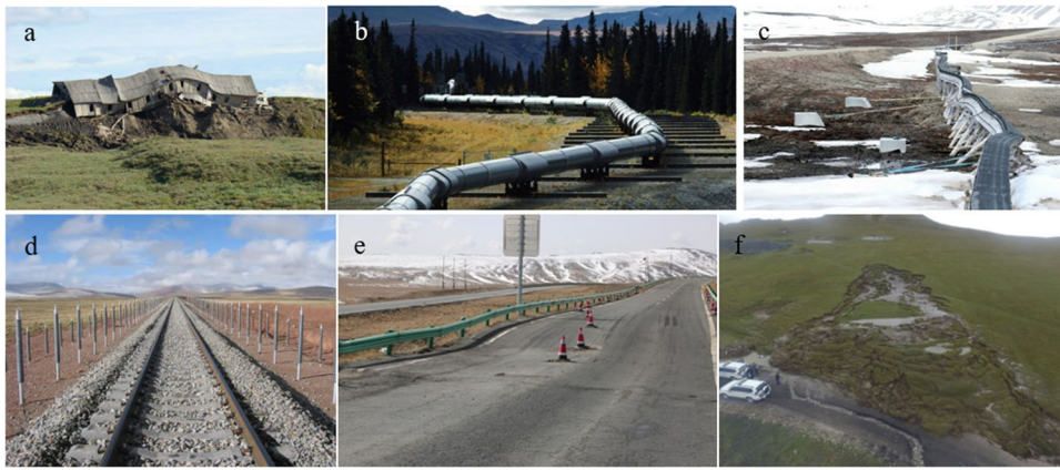
Fig. 6 Different types of infrastructure damages due to permafrost degradation. a Damaged army barracks on the Yenisei River, Russia (photo by Zhang Ze), b damaged roads in northern Canada (photo by Zhang Ze), c Trans-Alaska pipeline, Alaska, in the Arctic (photo by Kwaisi France), d the Qinghai-Tibet Railway, e highway and other roads at risk of land subsidence (photo by Tai Bowen), f thaw slumping on the QTP (photo by Luo Jing).
