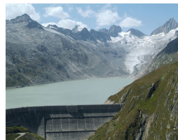
Hydropower station fed by ice-snow (clean energy) (SDG 7, 12)
