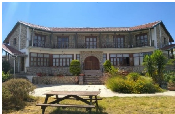
Fig. 10 Erson Hoca's Organic Farm Hotel—Limnitis. Example of reinforced concrete construction.
