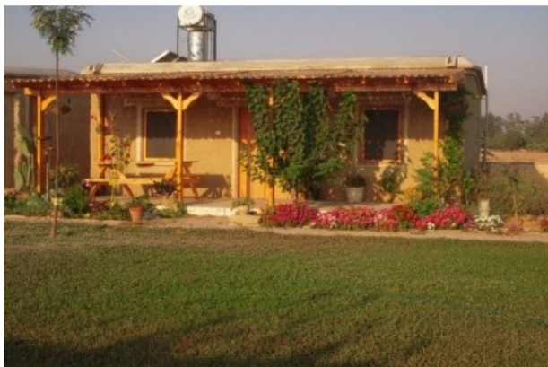
Fig. 7 Ay Phodios Guest House—Komikibir. Example of an adobe structure.
