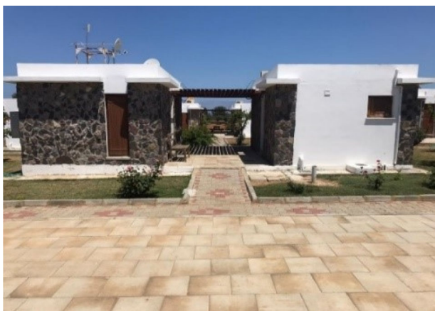
Fig. 8 Karpasia Natura Guest House—Risokarpaso. Example of reinforced concrete construction.
