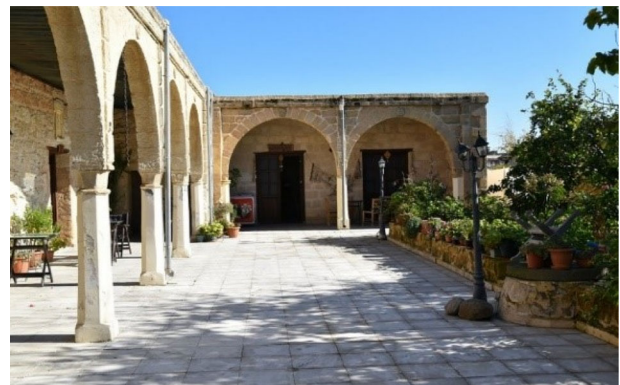
Fig. 14 Revaklı Ev Guest House. An example of a portico and arched structure—Risokarpaso.
