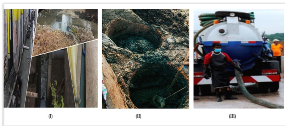
Fig. 3 Shows some on-site sanitation emptying practices in Khulna. (I) On-site sanitation systems discharging untreated effluent into public drains; (II) Manual emptiers in operations; and (III) Motorised on-site sanitation emptying trucks discharging to treatment plant.
