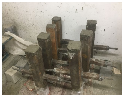
(b) Concrete was filled in the chord
