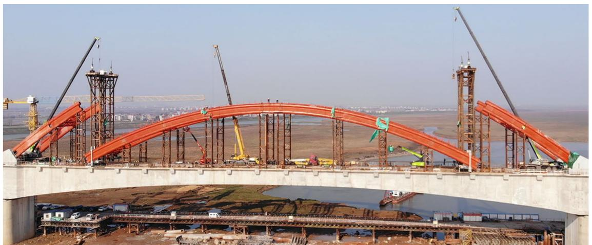
**Figure 11.** Construction of the low-level assembly.
