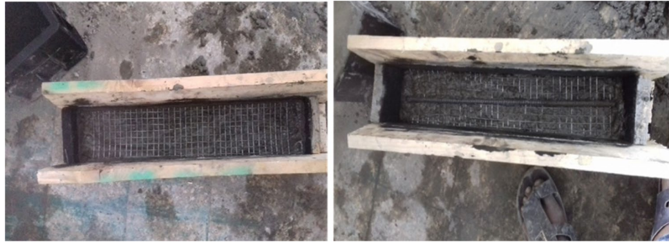
Figure 6. Casting of ferro concrete beam model using welded square wire mesh.
