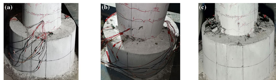
Figure 8. The state of the UHPC socket throughout the test. (a) Fully developed cracks. (b) Concrete spalling. (c) Final failures state.
