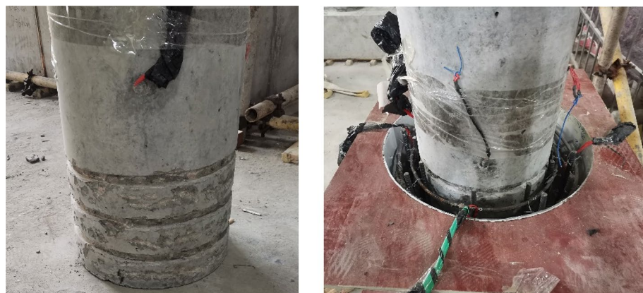
Figure 3. The grooved surface at the bottom of the column.
