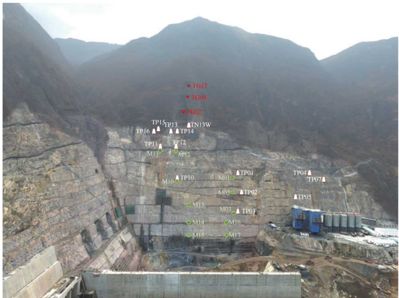
Figure 7. Distribution of effective monitoring points on the left bank slope.
