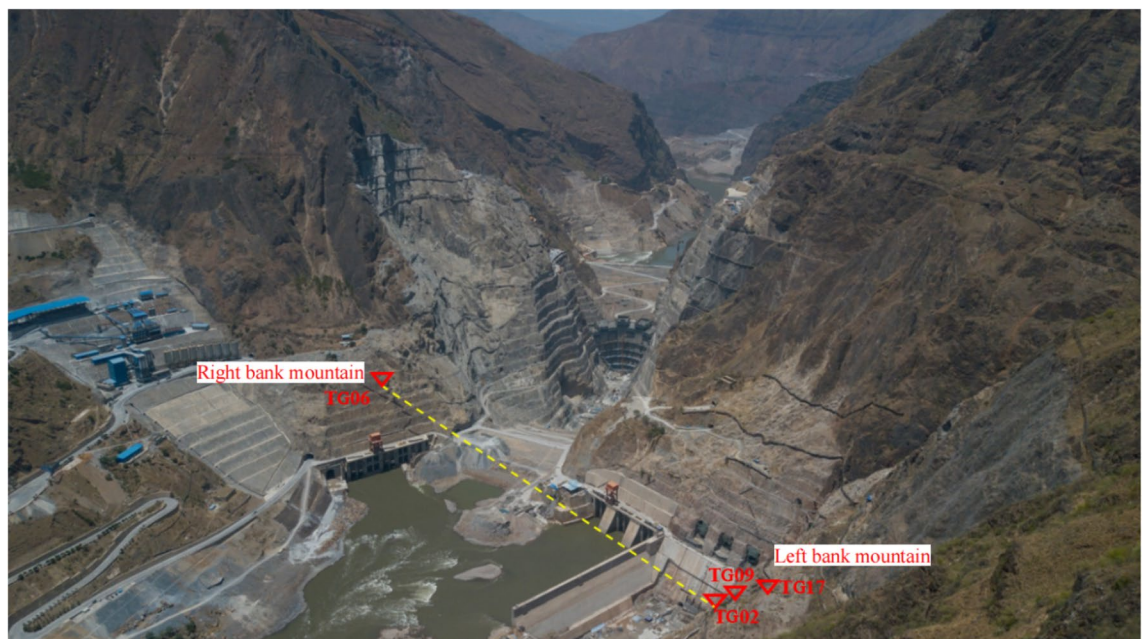
Figure 6. Distribution of mountain valley deformation monitoring points on both sides of water cushion pond in flood tunnel.
