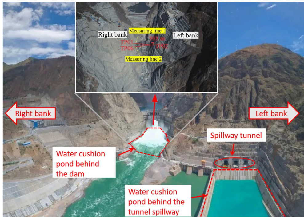
Figure 21. Location of water cushion ponds on the back side of the dam.
