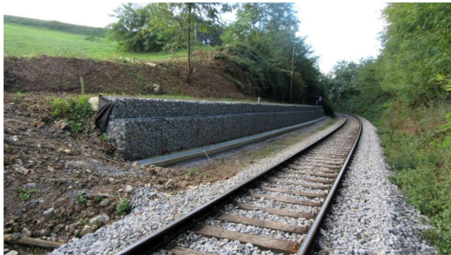
Figure 14. Picture of the retaining wall structure.
