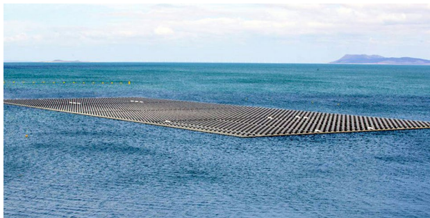
Figure 8. Floating PV Power Plant at Sobradinho hydroelectric power plant reservoir. to Springer Nature exclusively under CC BY SA for this study 63 .
