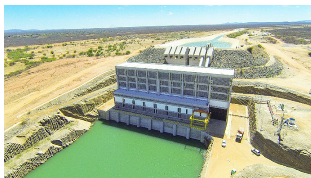
Figure 4. Pumping station EB-1. Source: Brazil---Ministry of National Integration/Disclosure.
