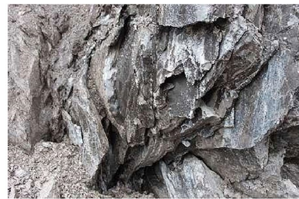
(b) Freeze–thaw toppling failure
