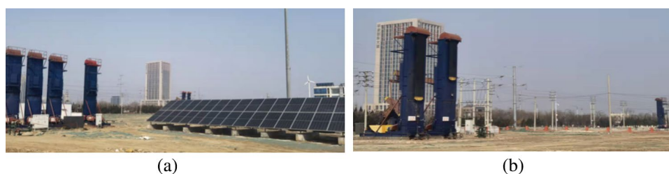
Figure 4. Test site of the DXX11 well group. (a) Partial panorama of the well site; (b) Participants in testing 4 wells.
