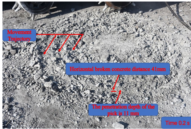
Figure 14. Result of concrete breaking by new shaft tunneling machine under optimum drum rotation speed.
