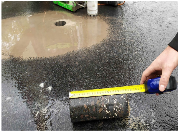
Figure 2. Core sample taken with the use of a hydraulic drilling rig.
