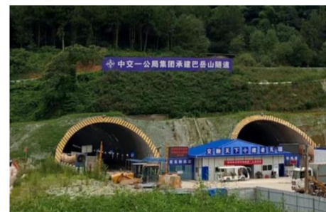
(b) The Bayue Mountain Tunnel entrance
