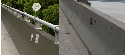
Figure 2. Concrete base with a height of 81 cm.
