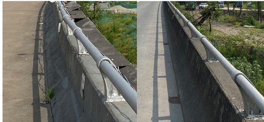
Figure 3. Concrete bases with heights of 63 cm and 68.5 cm.
