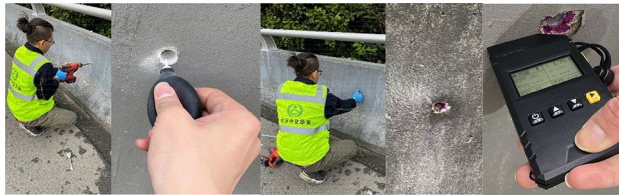
Figure 5. Detecting the depth of concrete carbonation.
