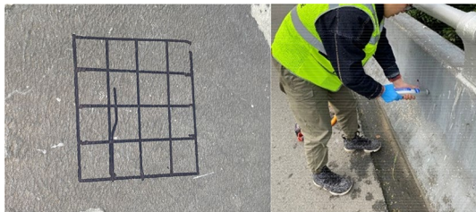
Figure 4. Detection of concrete strength using rebound method.
