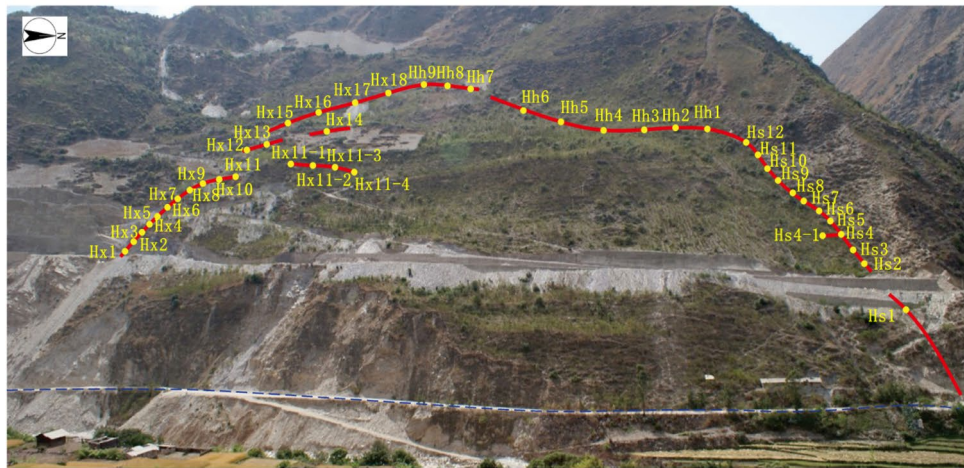
(a) Crack location distribution
