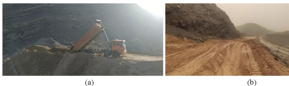
Figure 19. Loess backfilling on the slope: (a) Slope dumping of loess; (b) Slope top covering with loess.
