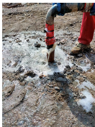
Figure 17. Filling boreholes with composite colloid in the field.
