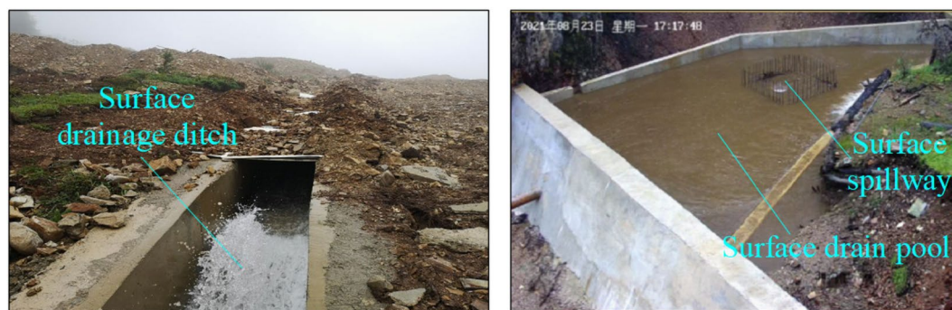
(a) Surface flood control by intercepting ditch
