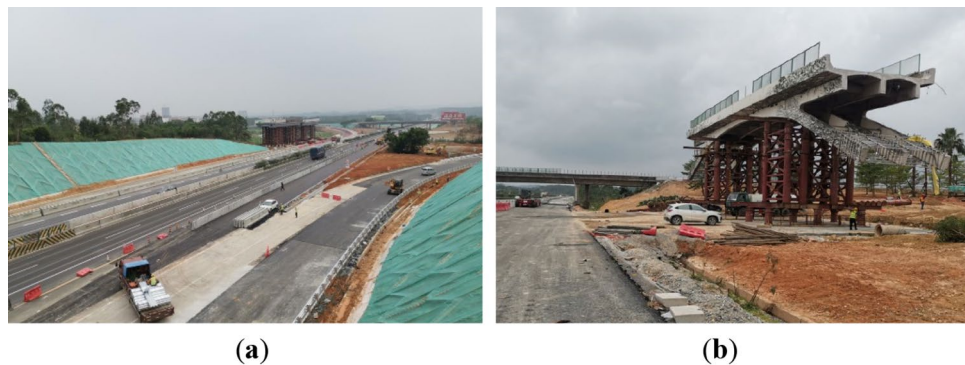
Figure 18. Photograph of (a) temporary transit route (b) temporary storage area.
