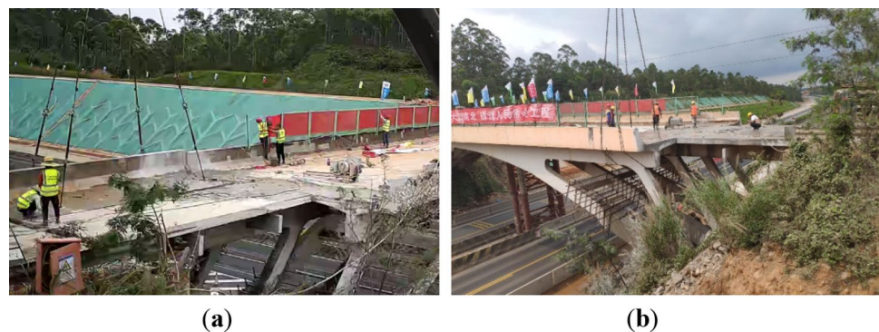
Figure 14. Hoisting of pre-cut bridge segments (a) outer segment 5-2 (b) inner segment 5-1.
