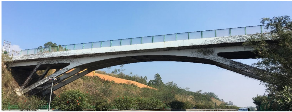
Figure 7. Photograph of the rigid-frame arch across the highway.
