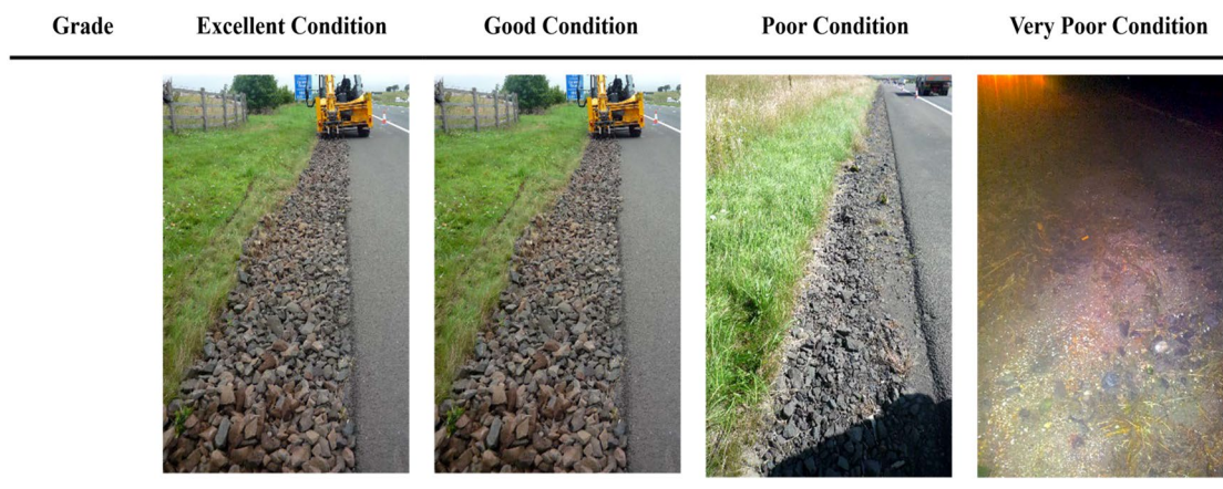
Figure 3. Visual representation of HFD conditions observed in the UK 15 . The excellent condition was as a newly constructed HFD, and the good condition had superficial defects but no obvious fouling 15 . The poor condition had moderate to high levels of fouling (i.e., part of the stone aggregate at the surface may not be visible at some angle), and the very poor condition possessed extreme foulants (i.e., the stone aggregate at the surface was not visible) 15 .
