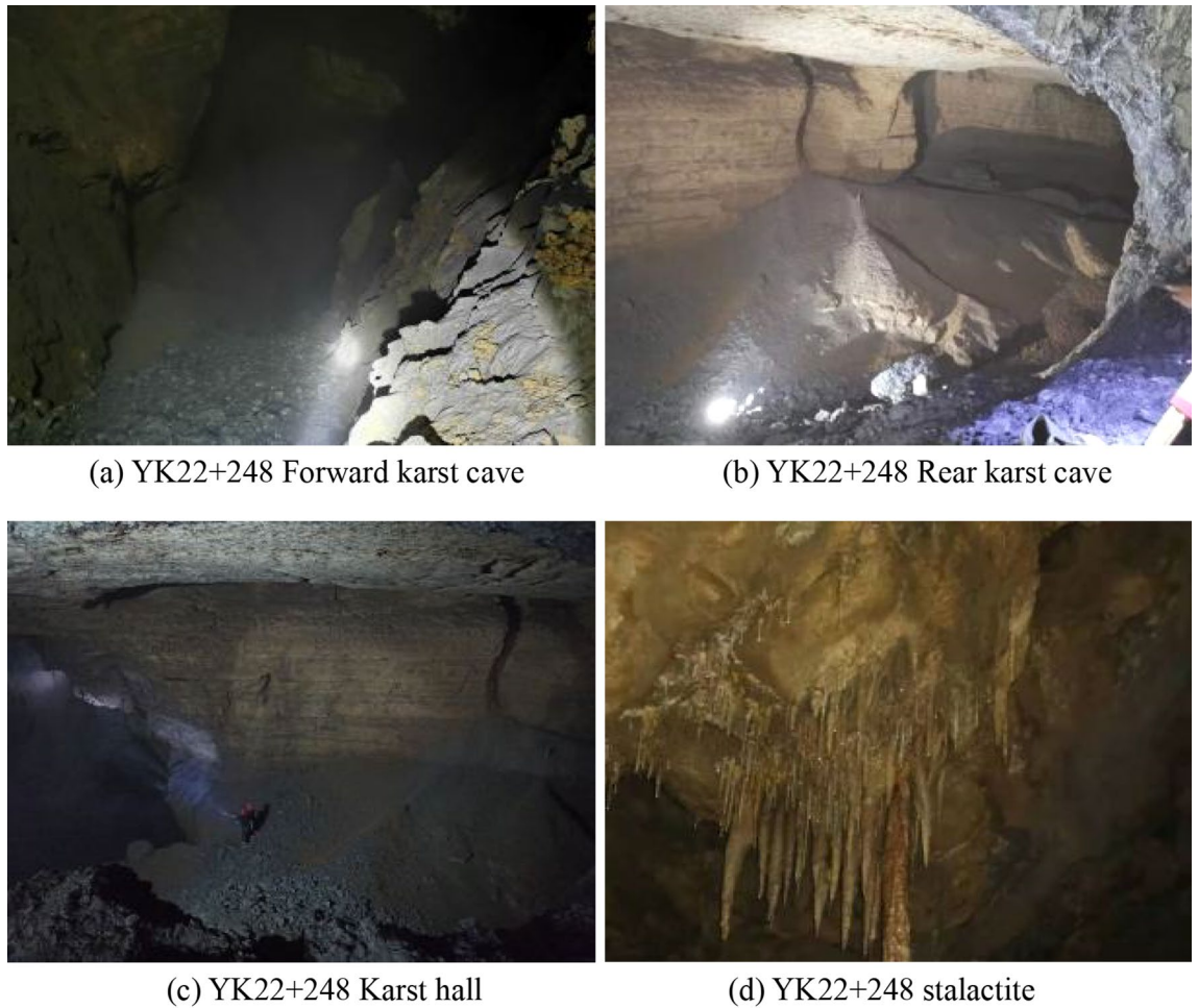
Figure 11. Karst cave in right tunnel.
