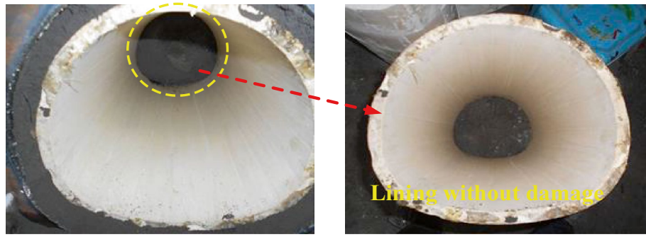
Figure 26. Lining without damage.
