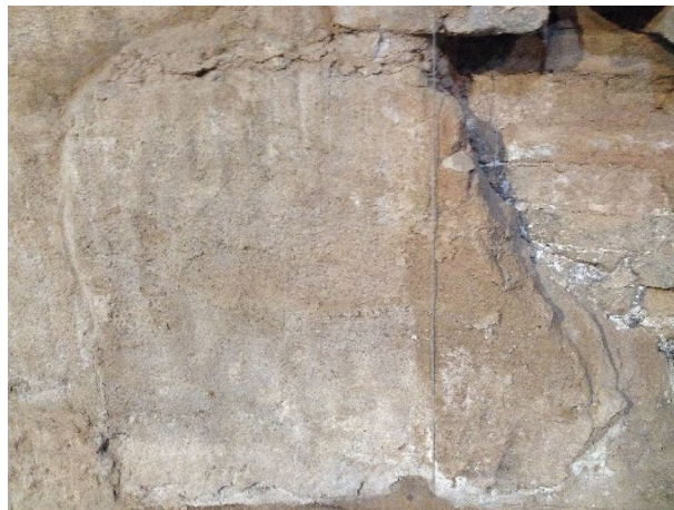
Figure 1. Salt precipitation on the surface of the site.
