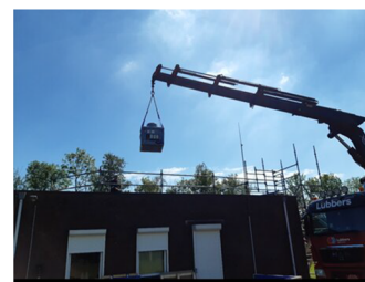
(b) Sensor being lifted into position.
