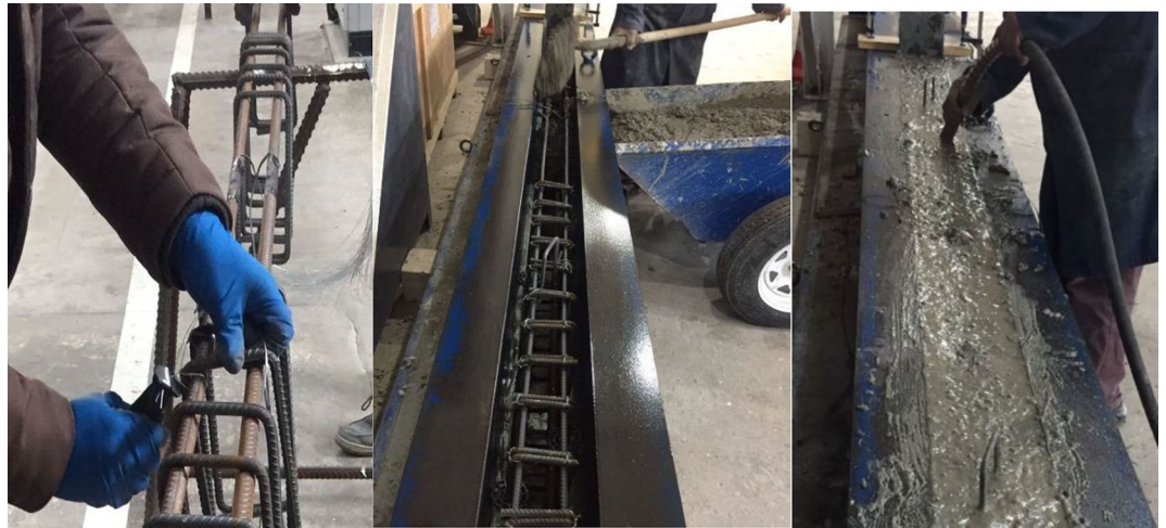
Figure 6. Construction of the Large-Scale Reinforced Beam.
