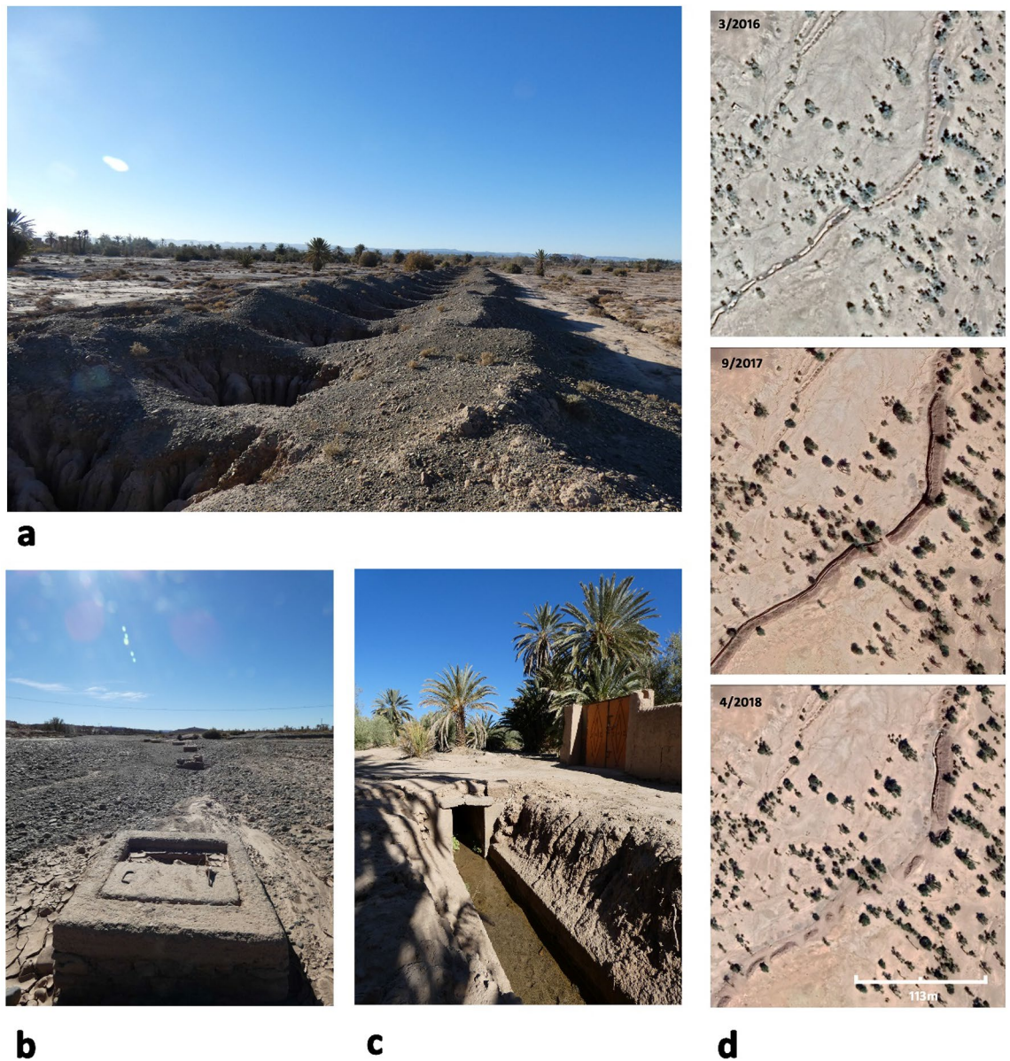
Figure 8. (a) Line of khattara shafts on the ground. (b) Line of shaft revitalised with concrete. (c) Water flowing from outlet lined with concrete. (d) Imagery showing stages of revitalisation of khattara. Photographs taken by Makovics and Rayne November–December 2022. Google Earth Pro map data: 2016 CNES/Maxar Technologies, 2017 MAXAR Technologies, 2018 MAXAR Technologies https://www.google.com/intl/en_uk/earth/versions/#earth-pro . Image prepared using GIMP 2.10.34 https://www.gimp.org/ .
