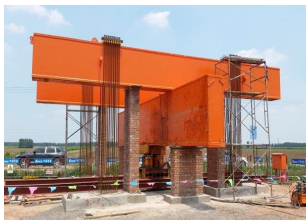
Figure 8. Photograph of the pile static load test equipment.
