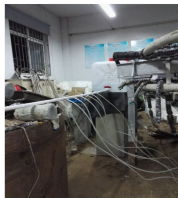
Figure 2. Layout of drainage system. (a) Schematic diagram of drainage structure; (b) drainage structure layout.
