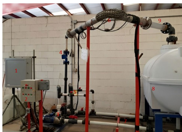
1. Data logger 2. Power control unit 3. Pumps 4. Flow meter 5. Control valve 6. Stainless steel 316 elbow with EFM pins 7. PVC pipes 8. Storage tank 9. Plexiglass section
