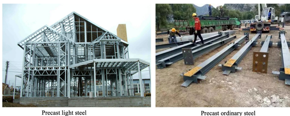
Figure 9. The two types of prefabricated components of Project C.
