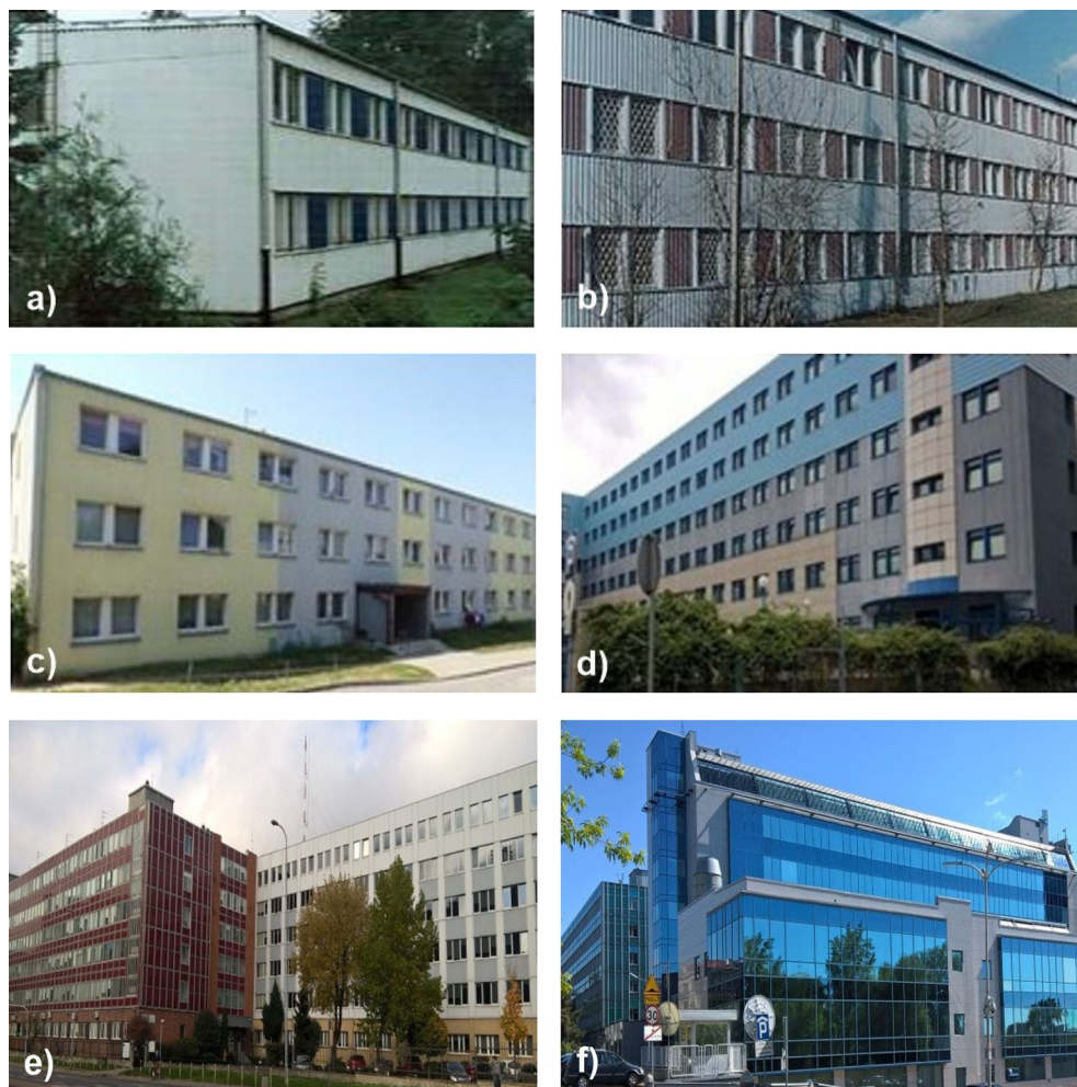
Figure 1. The tested buildings. Figure: (a) and (b) Typical “BERLIN” building, general view before renovation (Poland, Warsaw), (c) Current view of building type “BERLIN” no. 2 after correct renovation (enclosure and encapsulation) (Poland, Olsztyn), Buildings type “LIPSK” in Poland, Warsaw: (d) Building type “LIPSK” after similar renovation as building type “BERLIN” no. 2, (e) Poland, Warsaw, Complex of two connected buildings of type “LIPSK”, on the left, building no. 11 (red), on the left side, building no. 7 (white) on the right side, (f) Poland, Warsaw, Buildings type “LIPSK” after asbestos removal and change of façade. Inside, on the left – “LIPSK” without any modification, removal or replacement of construction products. Typical damages of “SOKALIT” are shown in Supplementary Information 1 and 2.
