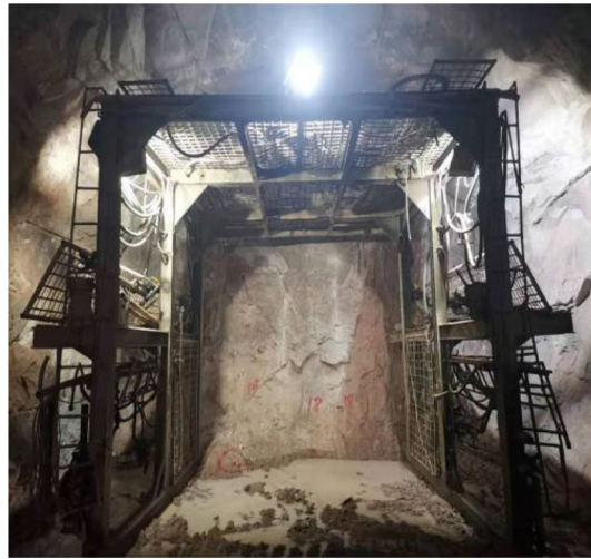
Figure 16. Excavation of the bench face at K2 + 077 in the field.
