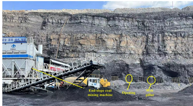
Figure 8. Auger mining engineering practice.
