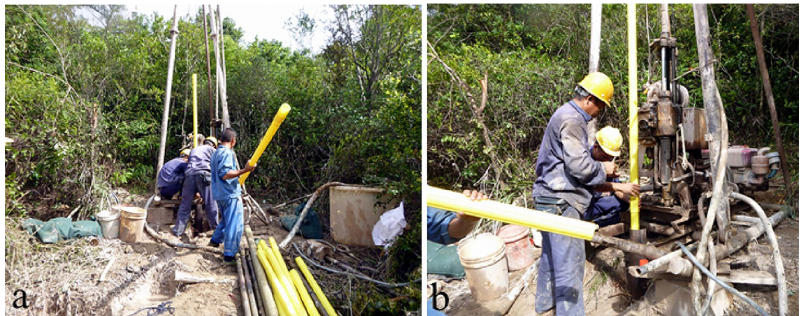
Figure 7. Installation of inclinometer pipe.
