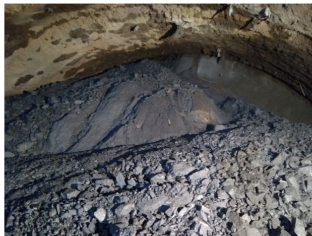
Figure 3. An example of the surrounding rock condition after excavation.
