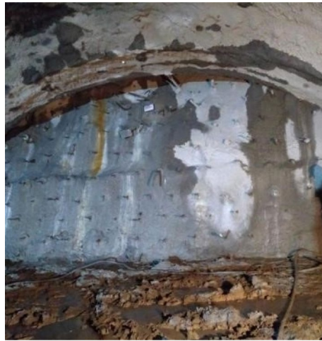
Figure 12. Example of the stabilized face.
