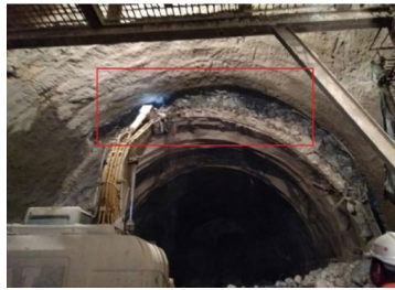
(a) Exchanging the steel arch frame at the intrusion section (DK80+390~410)
