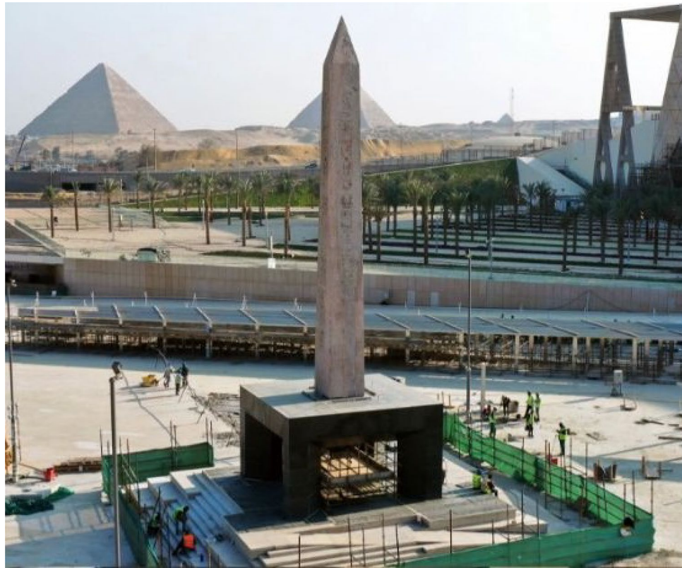
Figure 20. Obelisk after erection on its elevated platform.
