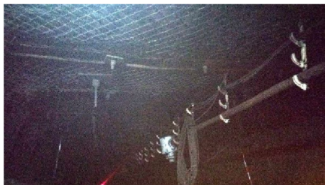
(a) Picture of roadway roof status
