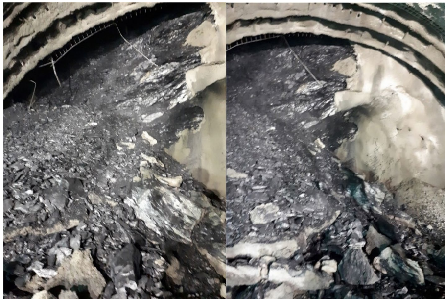
Figure 6. Tunnel face excavation view in the graphitic schist.
