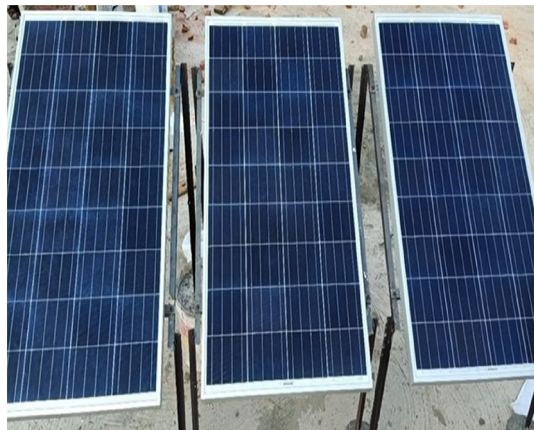
Figure 1. The Pv panels.
